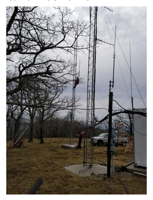
Danny (climbing) and Carl (on the ground). Replacing the 900Mhz- hard line for the repeater.
