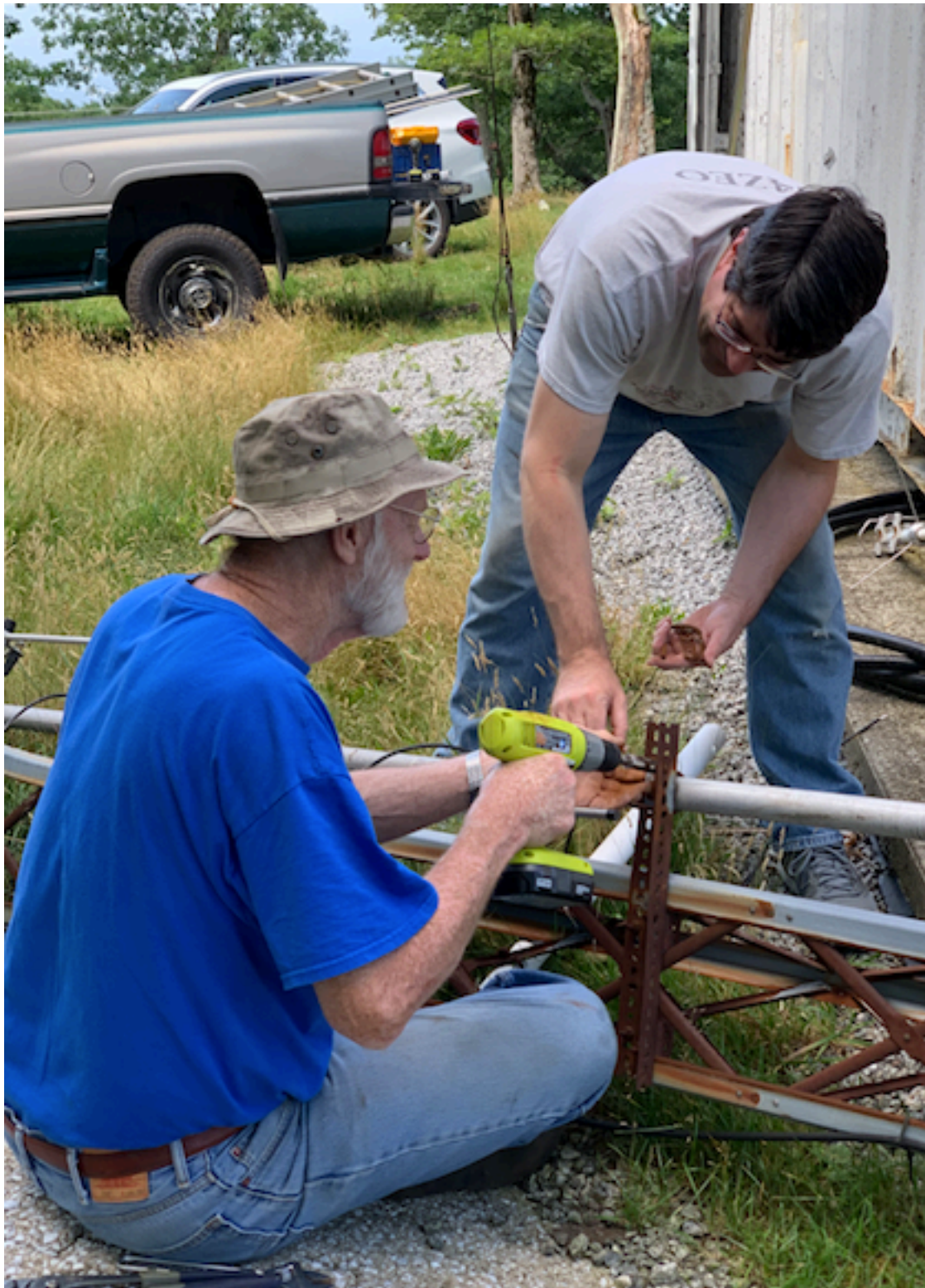
KW4EO and KJ4ZEO Repairing the Tower
