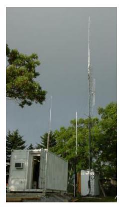
on a 40' tower. Should commercial power be lost, there is battery back-up which lasts 2 or 3 days, depending on usage. Transmitter power reduces to 10W during those occasions. The photo on the left shows the outside of the air-conditioned container housing the electronics, and affords a good view of the tower with its 2m antenna on the right.
