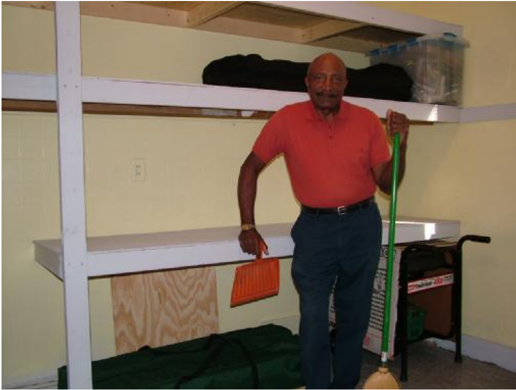
Ronnie Puts Finishing Touches on Storeroom
